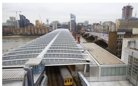
Scalo Solar @ScaloSolar World's largest solar-powered bridge opens in London.
